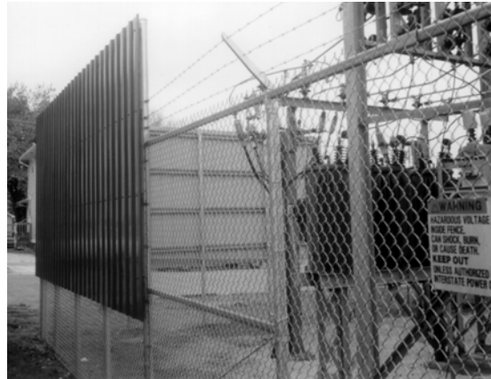
Figure H110A2-6 Solid section meeting TIA 2007-1 limits contact with close facilities, but does not comply with 2012 Rule 110A2 to have full vertical section solid
