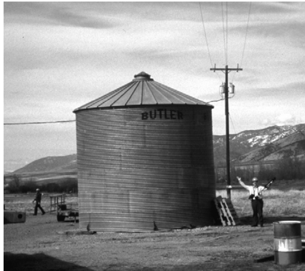
Figure H234F Grain bin clearance less than required by Rule 234F
