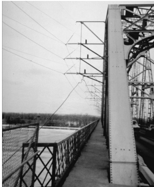
Figure H234D Attachment of conductors to a bridge
