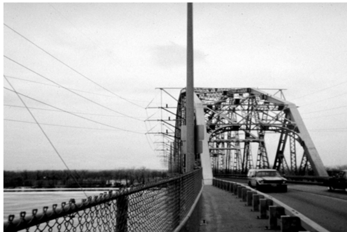
Figure H217A1c Power lines carried on bridge attachments
