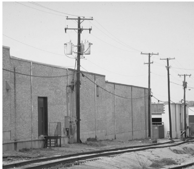
Figure H_T234-1_1 Transformer bushing and jumper clearance less than required by Table 234-1 and Rule 234J
