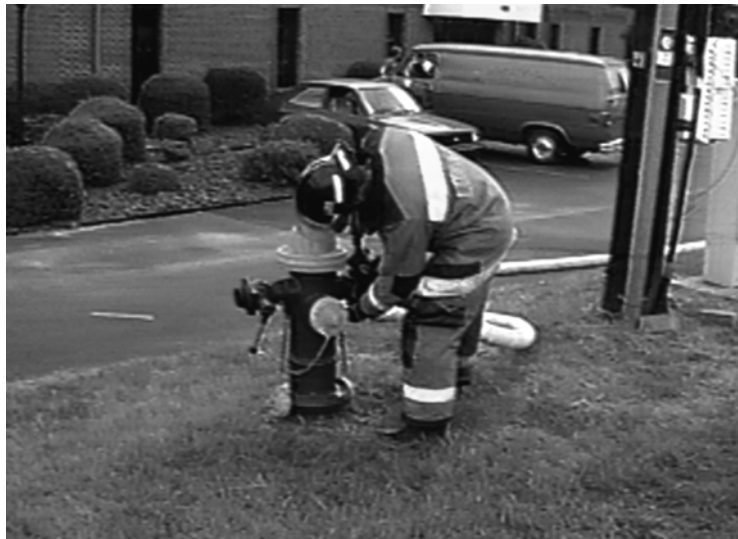
Figure H231-1 Fire hydrant with portable gate valve attached
