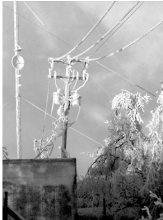
Figure H250B Ice on pole and supported facilities
