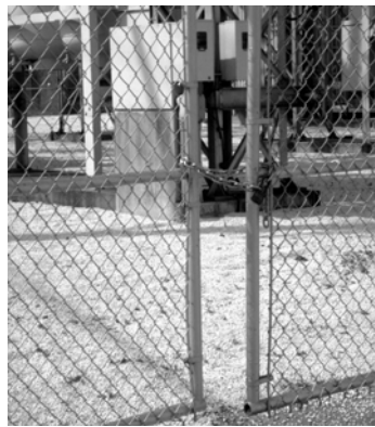
Figure H110A1-7 Supply station fence gate with too large a gap between panels
