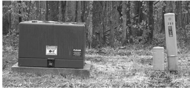
Figure H384C Power and communication pedestals requiring bonding
